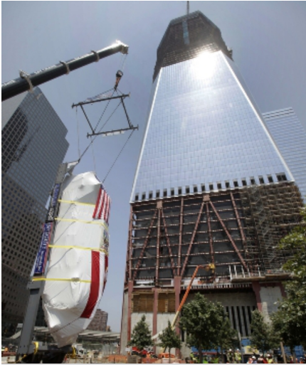
Baker team rigs Ladder Company 3 fire truck into National 9/11 Memorial & Museum
